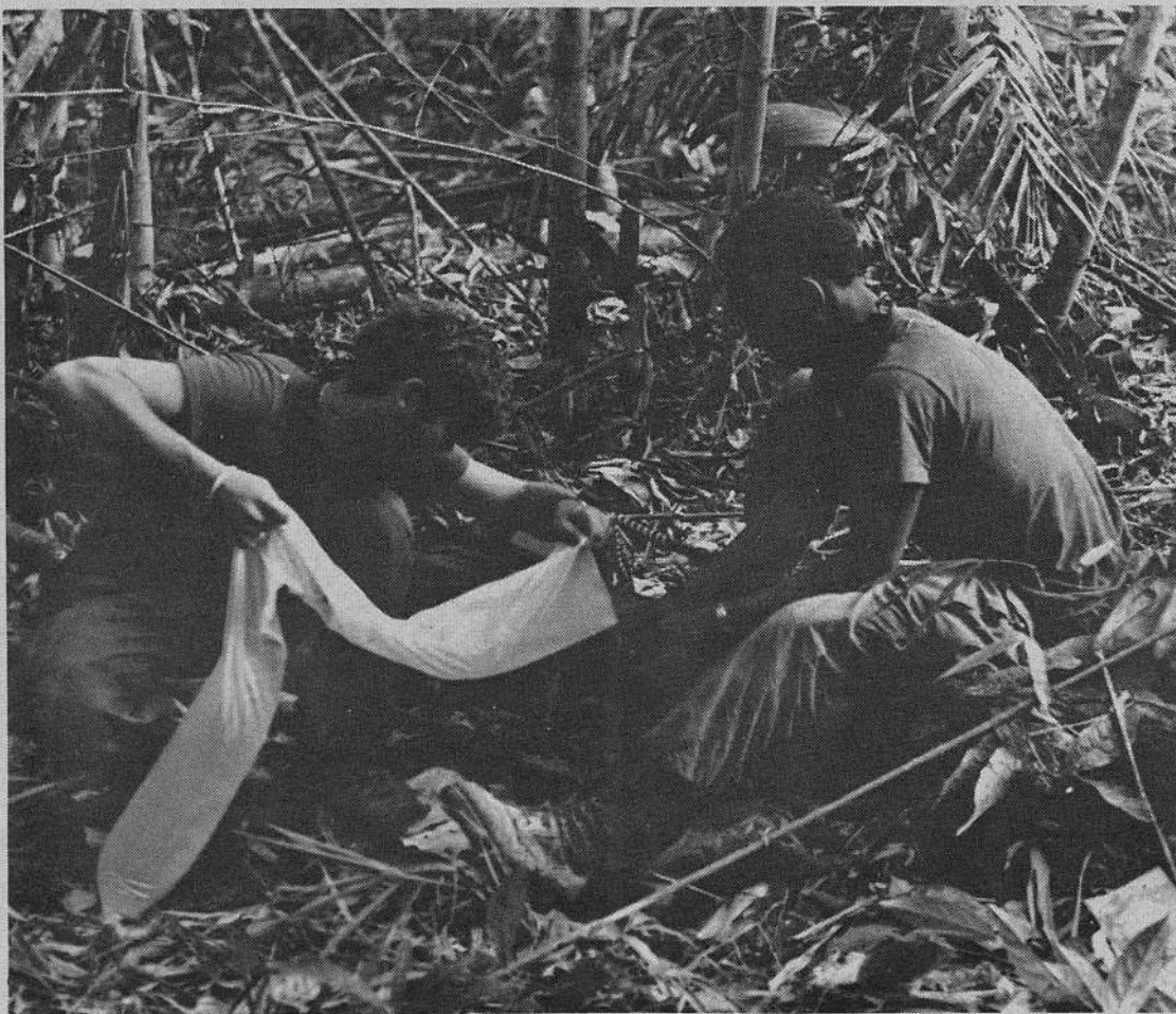
THEIR BAG -- Spec 4 Tony Katz, left, and PFC Howard Faulkner of HHC, 2nd Bn, 12th Cav, do their bit in building their new home--FSB 11 Bravo.
